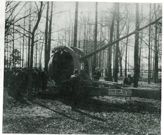
The tallest tree is lifted from the ground and lowered horizontally to be moved to the new location.
